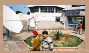
These HNS-built antennas, called very small aperture terminals (VSATs), were installed on the grounds of the Delhi stock exchange in 1997. They are part of a new VSAT network that links member brokers across India to facilitate securities trading, HNS leads the world in installing and operating VSAT networks.
